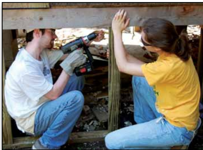
Ethan Gates and Alison Paetz putting in new floor joists.
