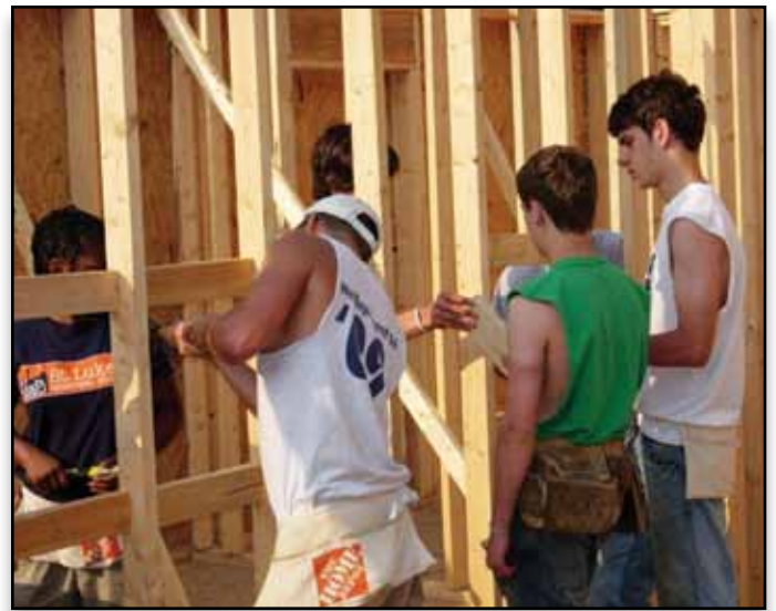
St. Paul's high school group framing a wall for cabinets in new housing (2006).
